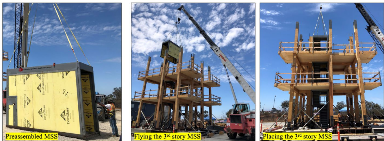
Figure 5: Installation sequence of modular stair system (MSS) unit with fire-rated shaft wall panels
