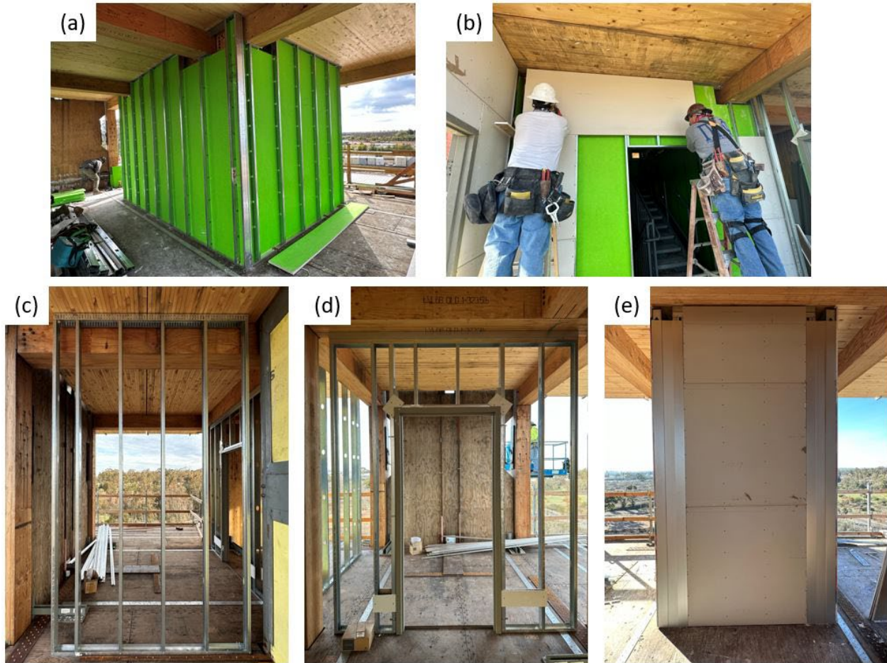
Figure 3: Interior wall construction: (a) shaft wall outline, (b) – (d) various wall junctions with gaps for vertical joints (not yet installed), (e) finished wall with corner joint assembly.
